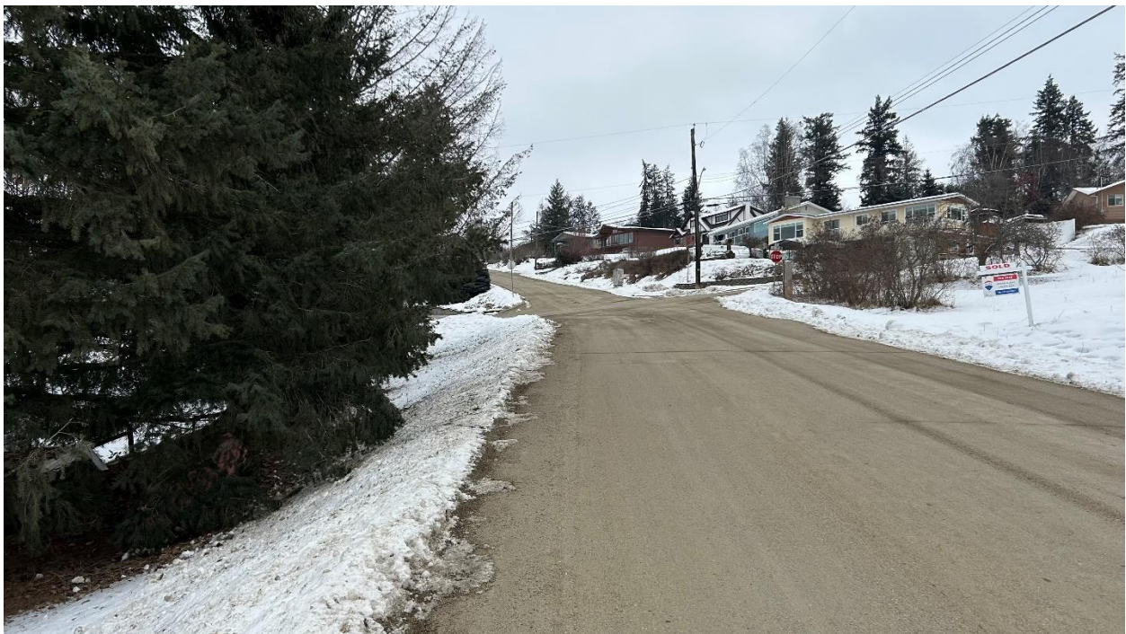
View of 13 Avenue SE from the SW corner of the subject parcel facing east.
