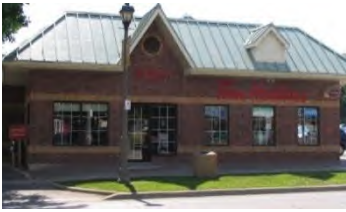
A good example of an interesting roof and a coordinated façade
