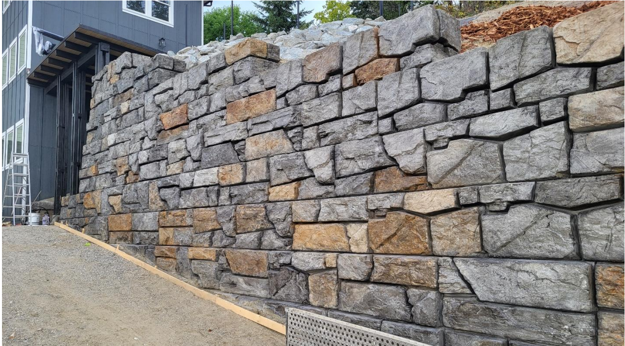
Photo 3: Existing Verti-block retaining wall on another property. The proposed Verti-block retaining wall along Auto Road SE is planned to have similar staining.
