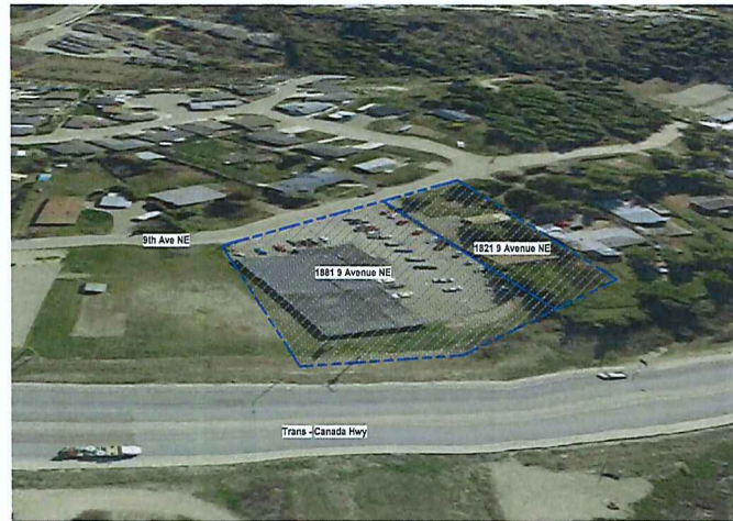
VIEW FROM NORTH
