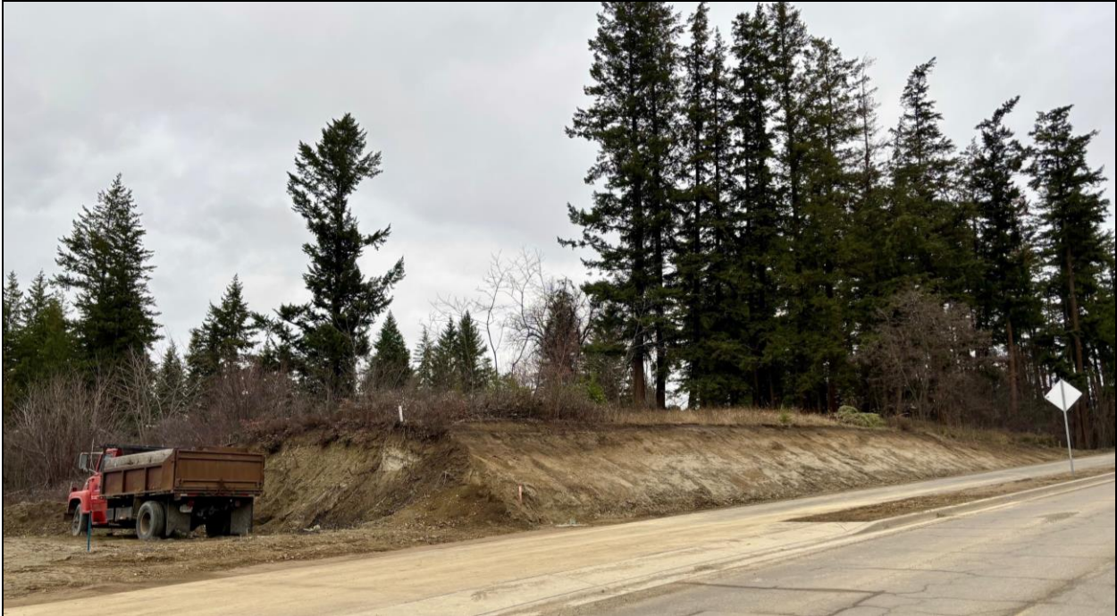
View northeast from 11 Avenue NE of subject parcel.
