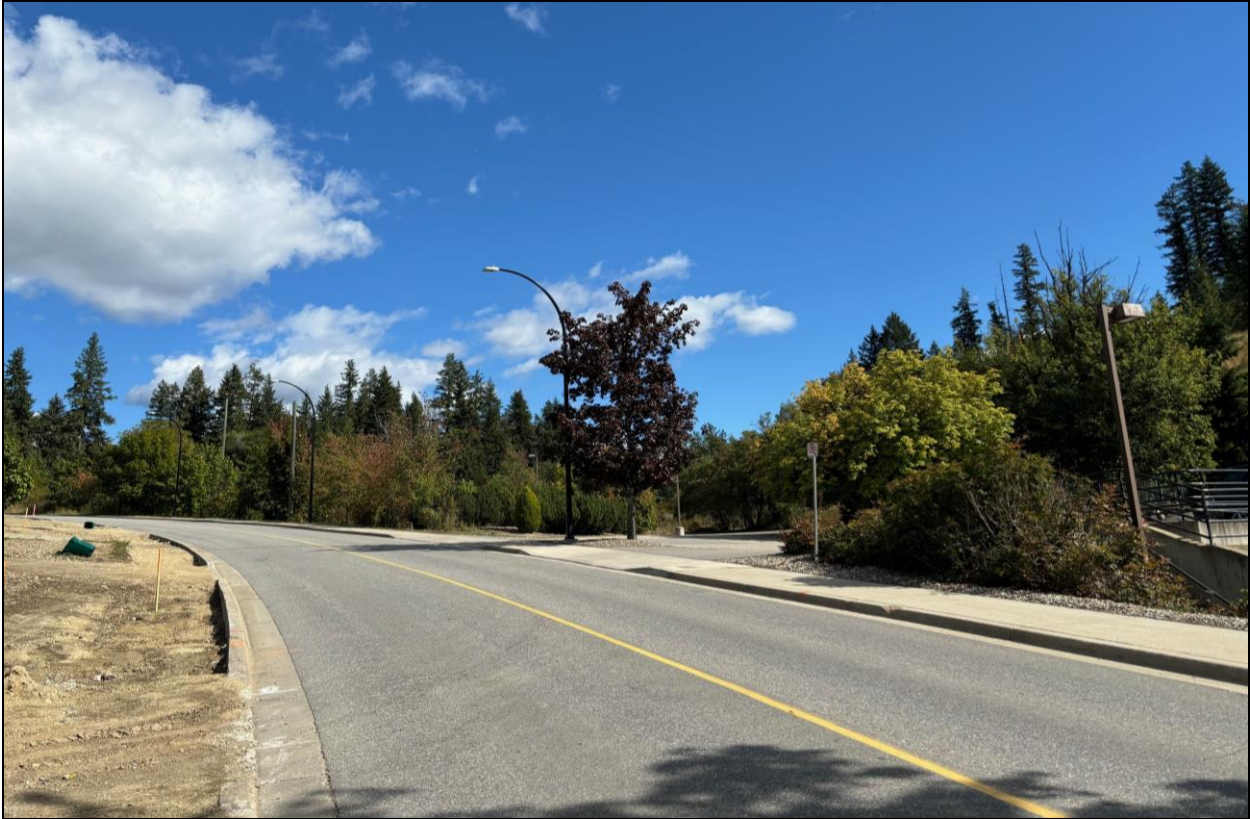
View of subject parcels from 16 Street NE looking northeast.
