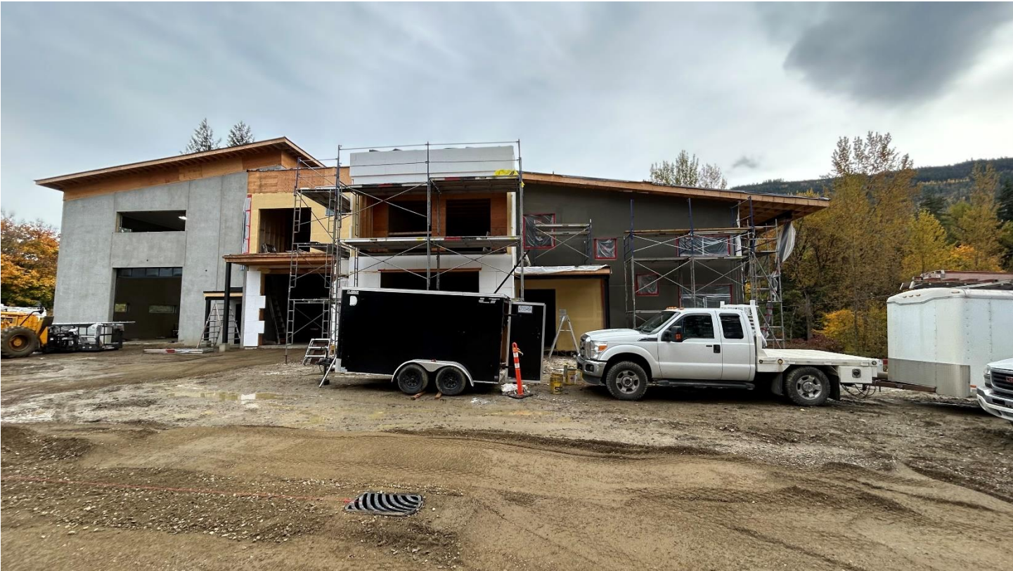
View of building currently under construction looking east from subject property.
