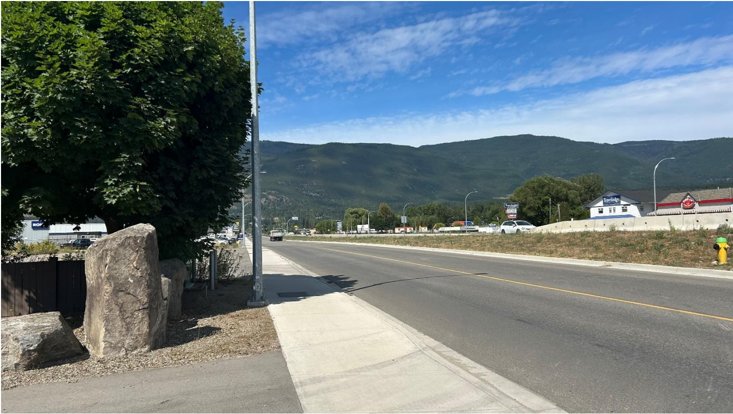
View of 10 Avenue SW looking northwest from 2270 10 Avenue SW.
