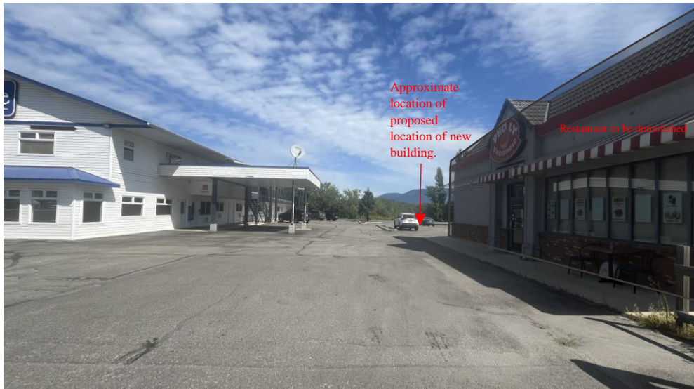
3. Looking north, towards the rear property line.
