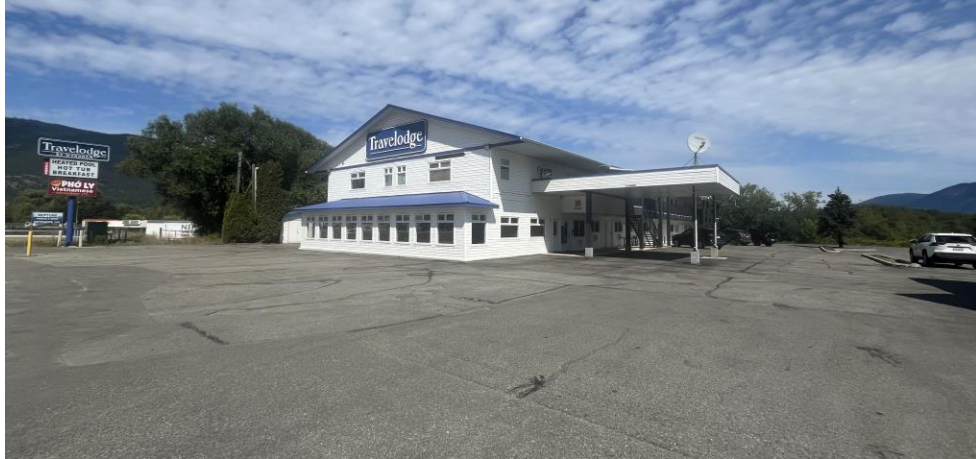
1. Looking northwest, towards existing motel.
