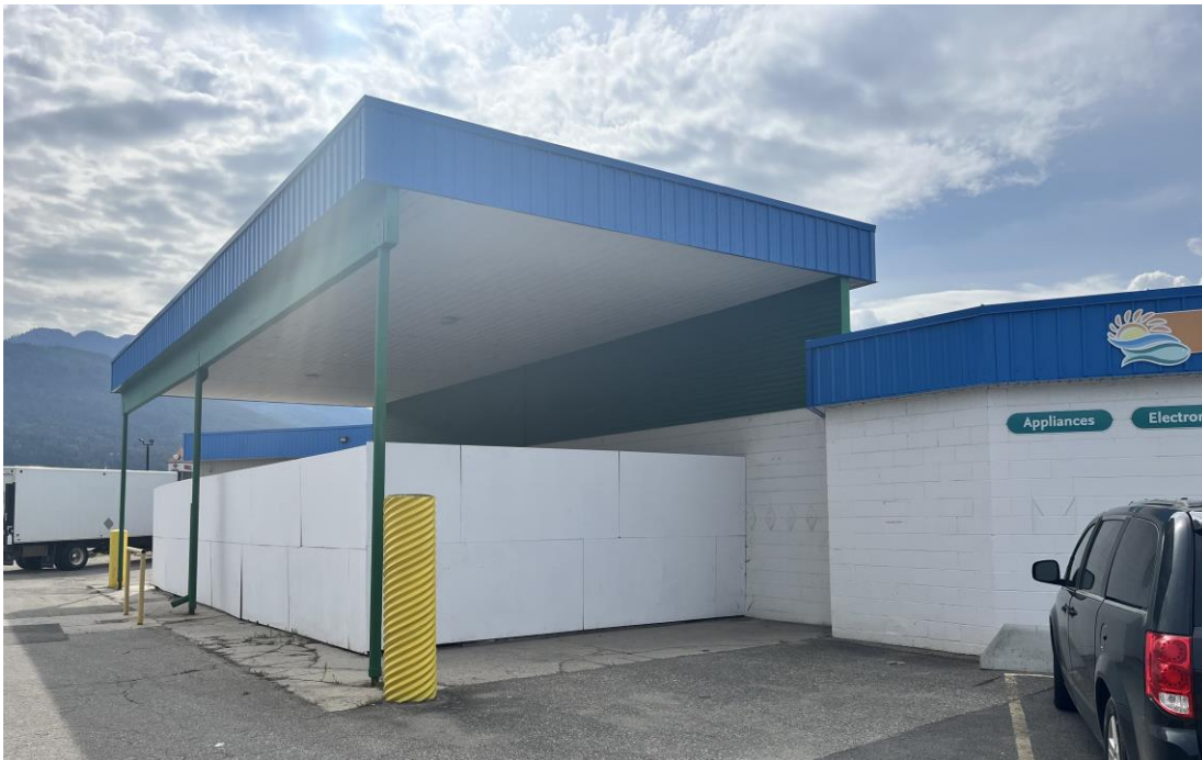
2. View of the open roofed area. Facing South.
