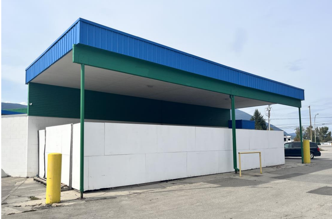
1. View of the open roofed area. Facing North West towards the front property line.
