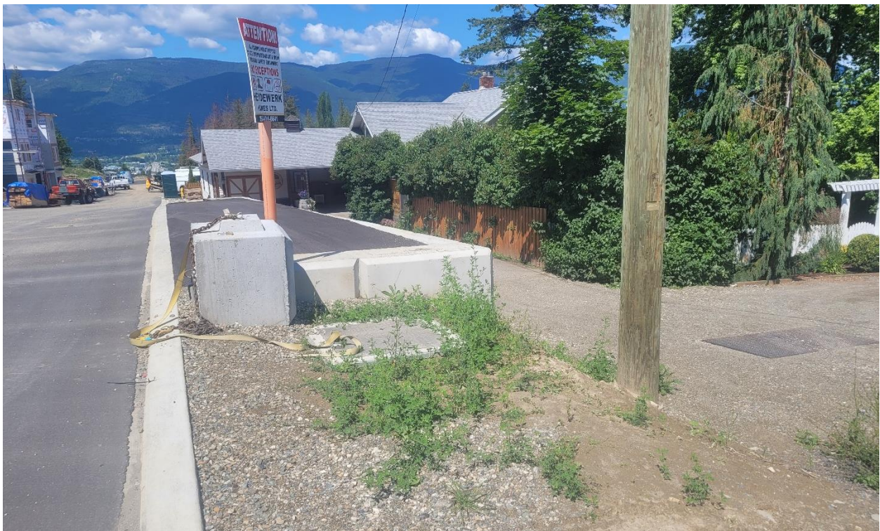
Photo 2: Parking area at top of Lock-Block retaining wall.
