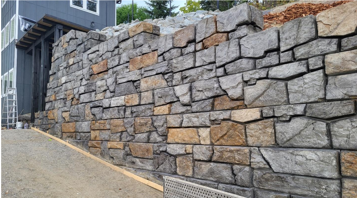
Photo 3: Existing Verti-block retaining wall on another property. The proposed Verti-block retaining wall along Auto Road SE is planned to have similar staining.
