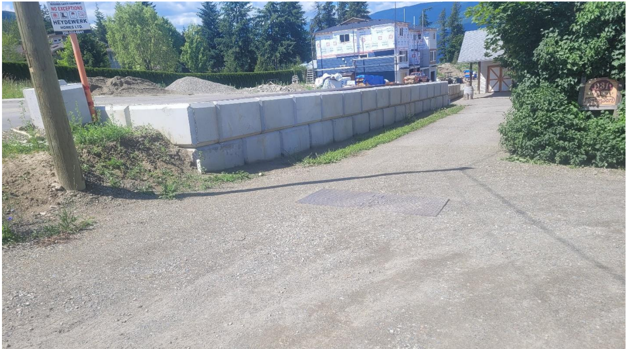
Photo 1: Lock-Block retaining wall along property line between 981 12 Street NE and 931 12 Street NE. Development Permit application proposes to install a privacy fence along the top of the retaining wall.
