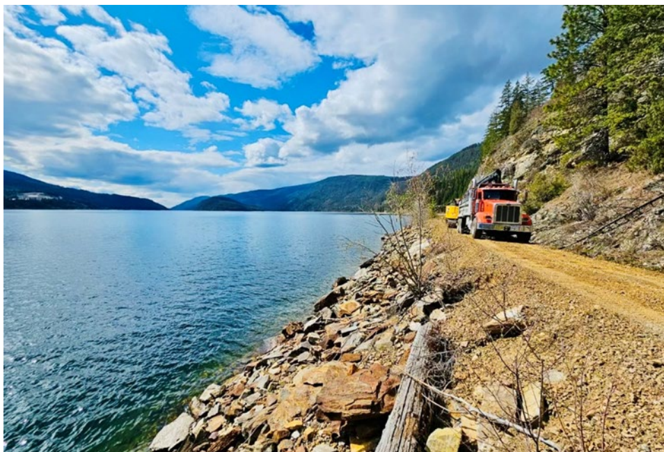
Shuswap North Okanagan Rail Trail Construction
