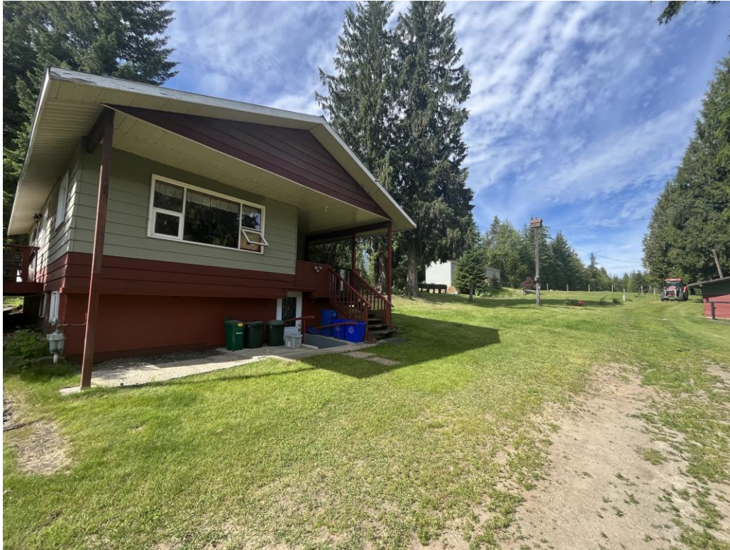
Looking southwest from the view of the barn/stables on subject property.
