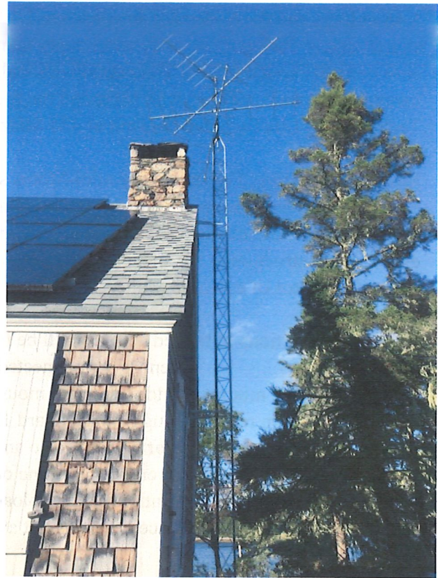
Motus station antennas mounted on a tower bracketed to a building. Photo: Northeast Motus Collaboration
