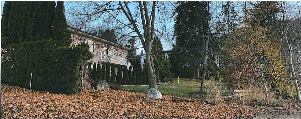
View southeast from greenway corridor, existing deck/stairs visible.
