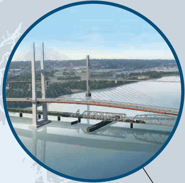
Pattullo Bridge Replacement Project
